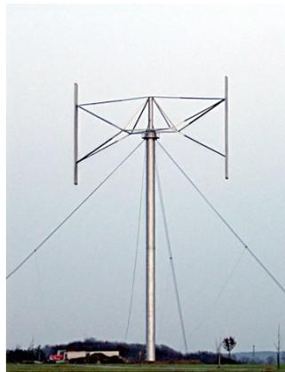
Fig. No. 06: Giromill type wind turbine<sup>[21]</sup>
